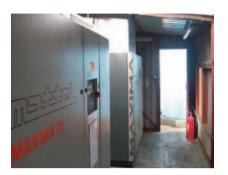
valve actuators and air driven motors. Prior to the data logging research, Petrochem Carless was using two 90kW Mattei compressors installed 12 years previously and was backed up by service support from the manufacturer.
