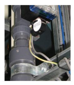
plant is a study in the use of level sensing technologies. Burkert 8110 vibrating level switches provide high and low level monitoring in the mould and resin mix tanks; its 8175 ultrasonic level transmitters look after the mix tanks and vessels linked to the pump sets, while type 8185 guided microwave level transmitters monitor the vacuum tanks.
